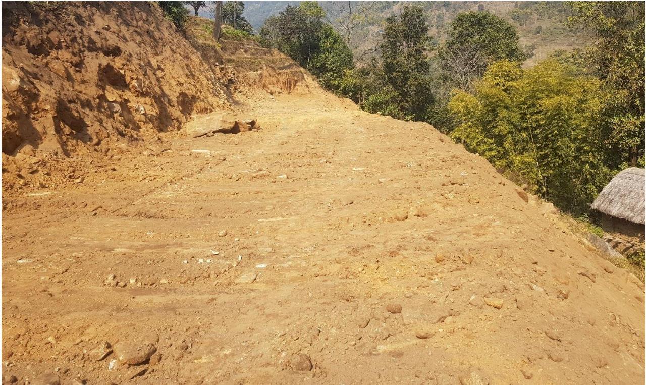
Figure 6.16: Track Widening for Headrace Pipeline Alignment
