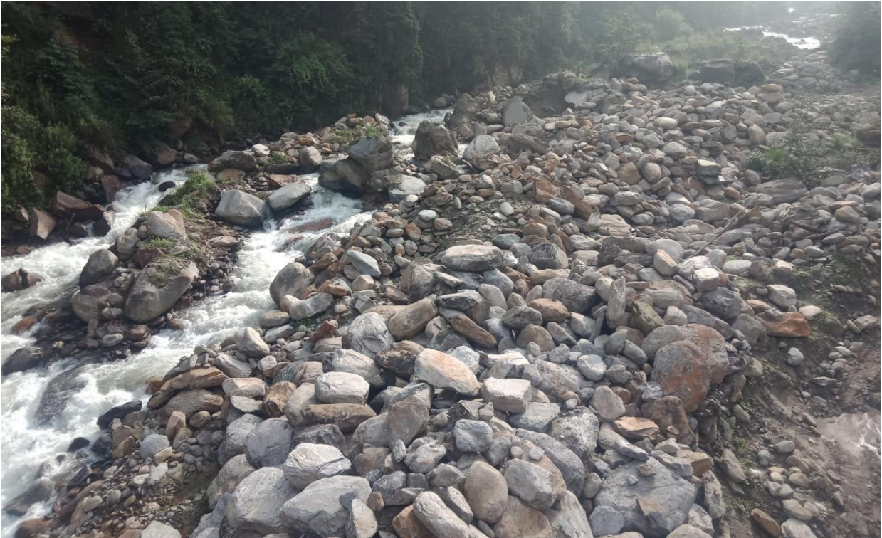
Figure 6.9: River training works upstream of headworks.
