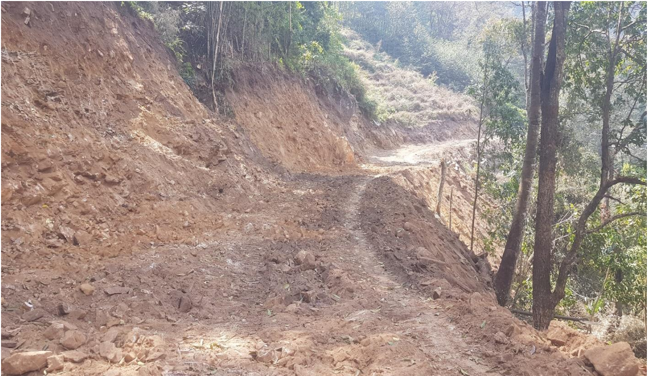
Figure 6.14:Track Widening for pipeline alignment.
