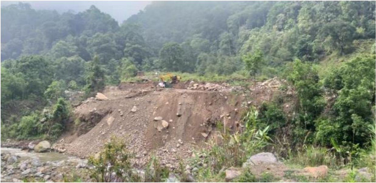
Figure 6.18: Powerhouse excavation work.
