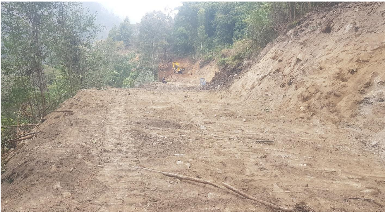
Figure 6.15: Track widening for waterway alignment.
