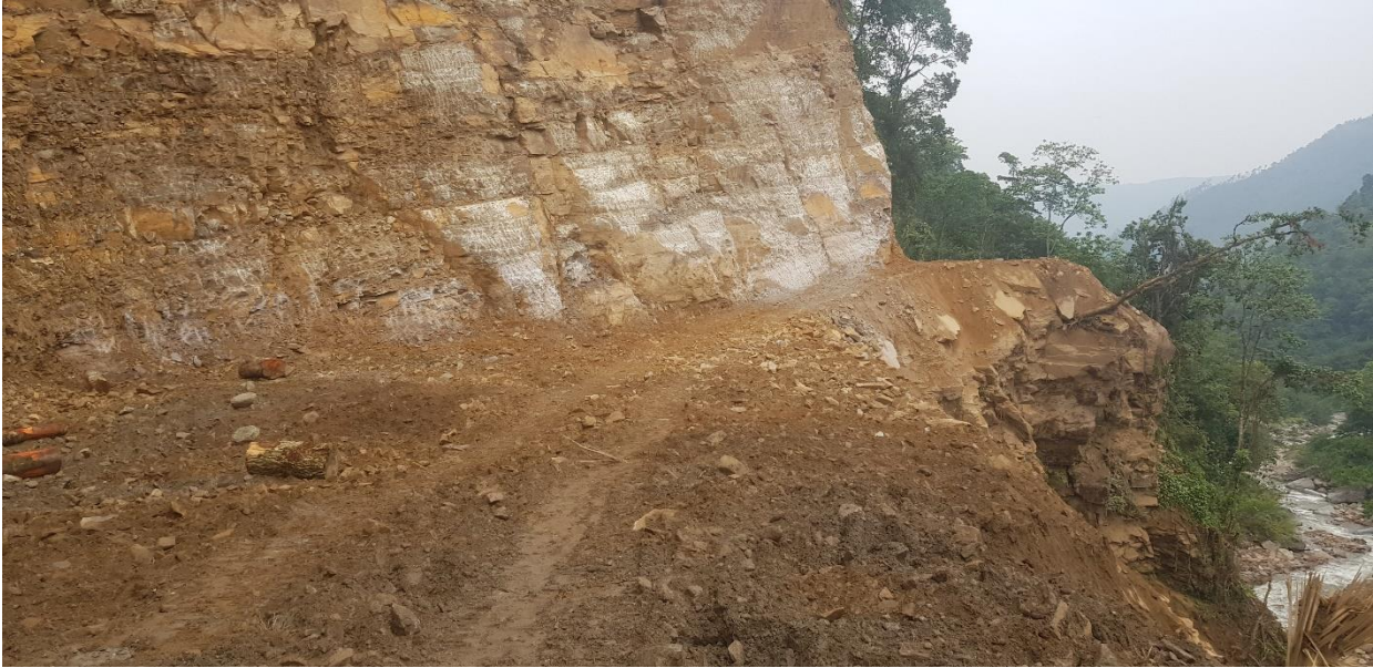
Figure 6.11:Track Widening for pipeline alignment after rocky cliff.
