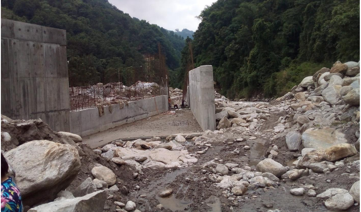
Figure 6.3: Undersluice upstream bay and divide wall.
