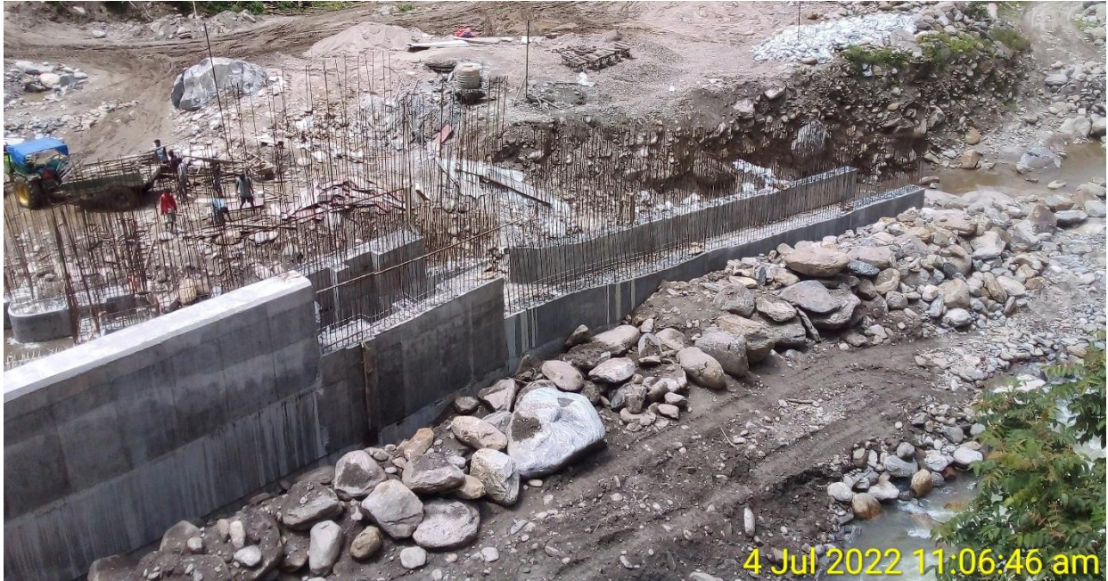
Figure 6.1: Undersluice slab concreting.
