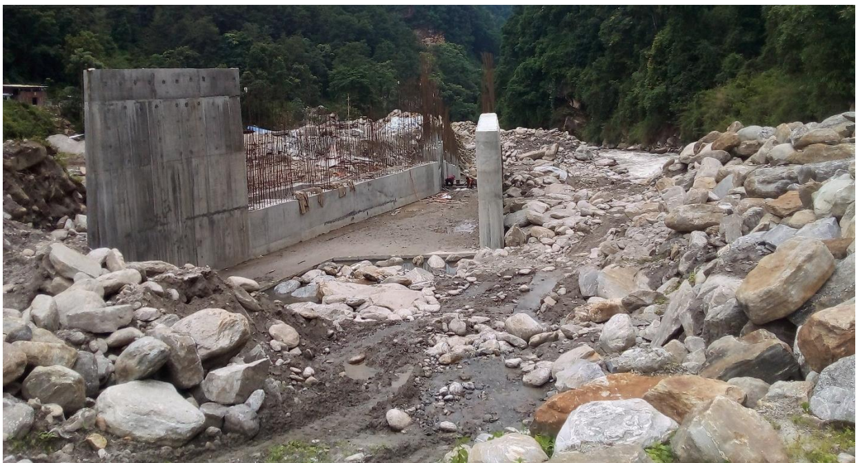
Figure 6.4: Guide wall and undersluice upstream slab from river side.
