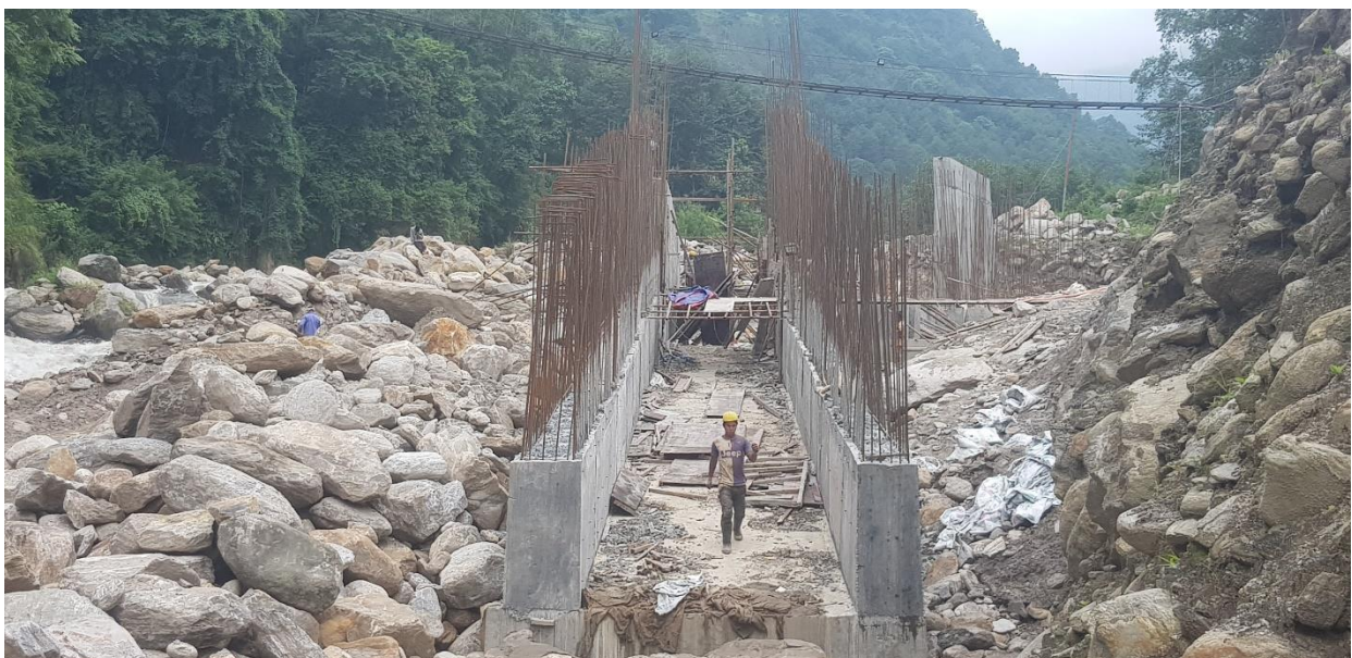
Figure 6.2: Formworks at Undersluice wall from downstream
