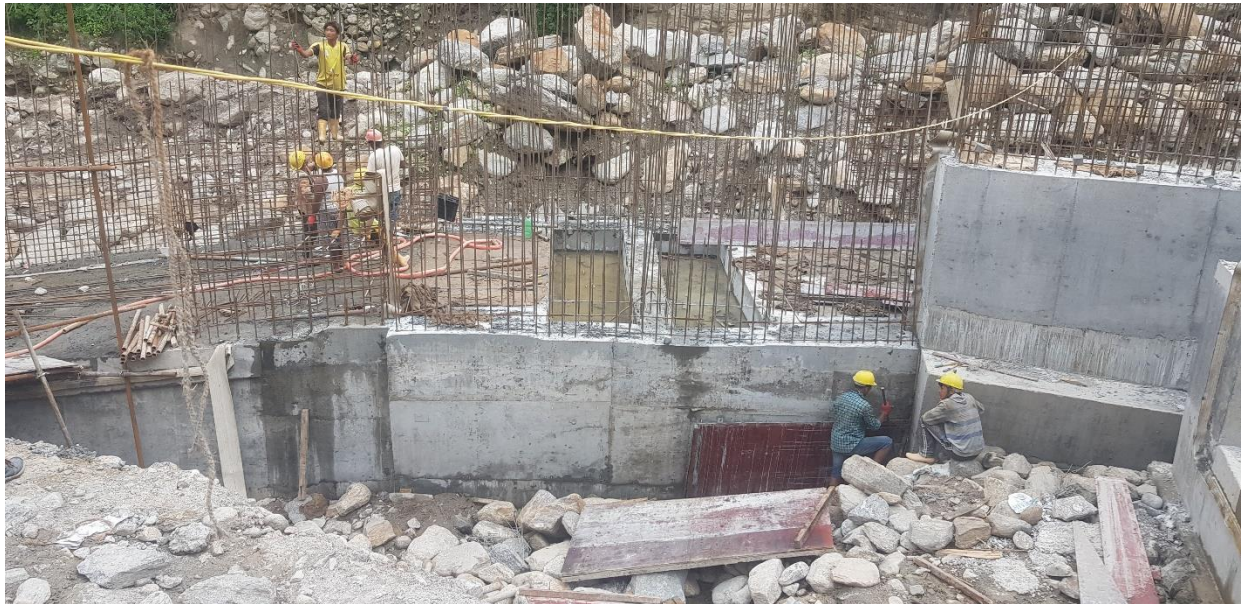
Figure 6.8: Gate grooves after concreting.
