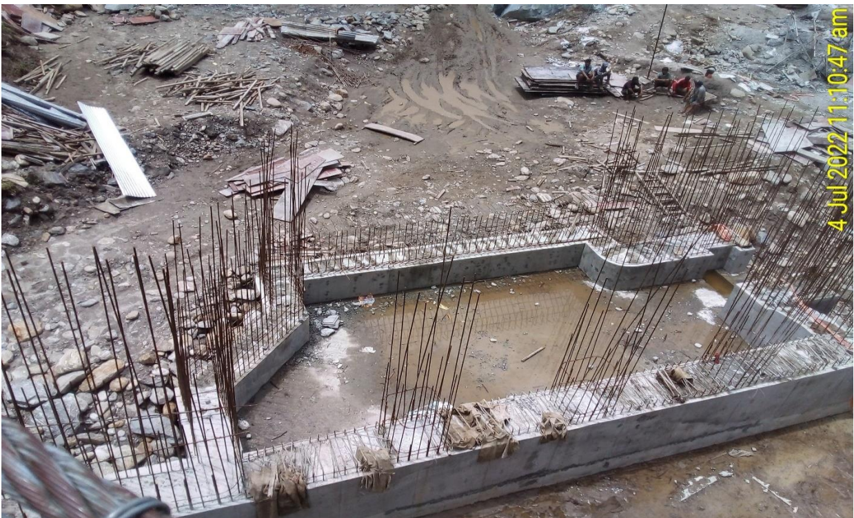
Figure 6.6: Intake, intake sluice and gravel trap area
