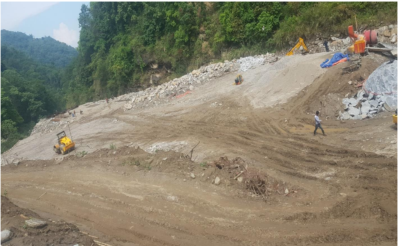
Figure 6.10: Gravel trap and desander inlet base preparation
