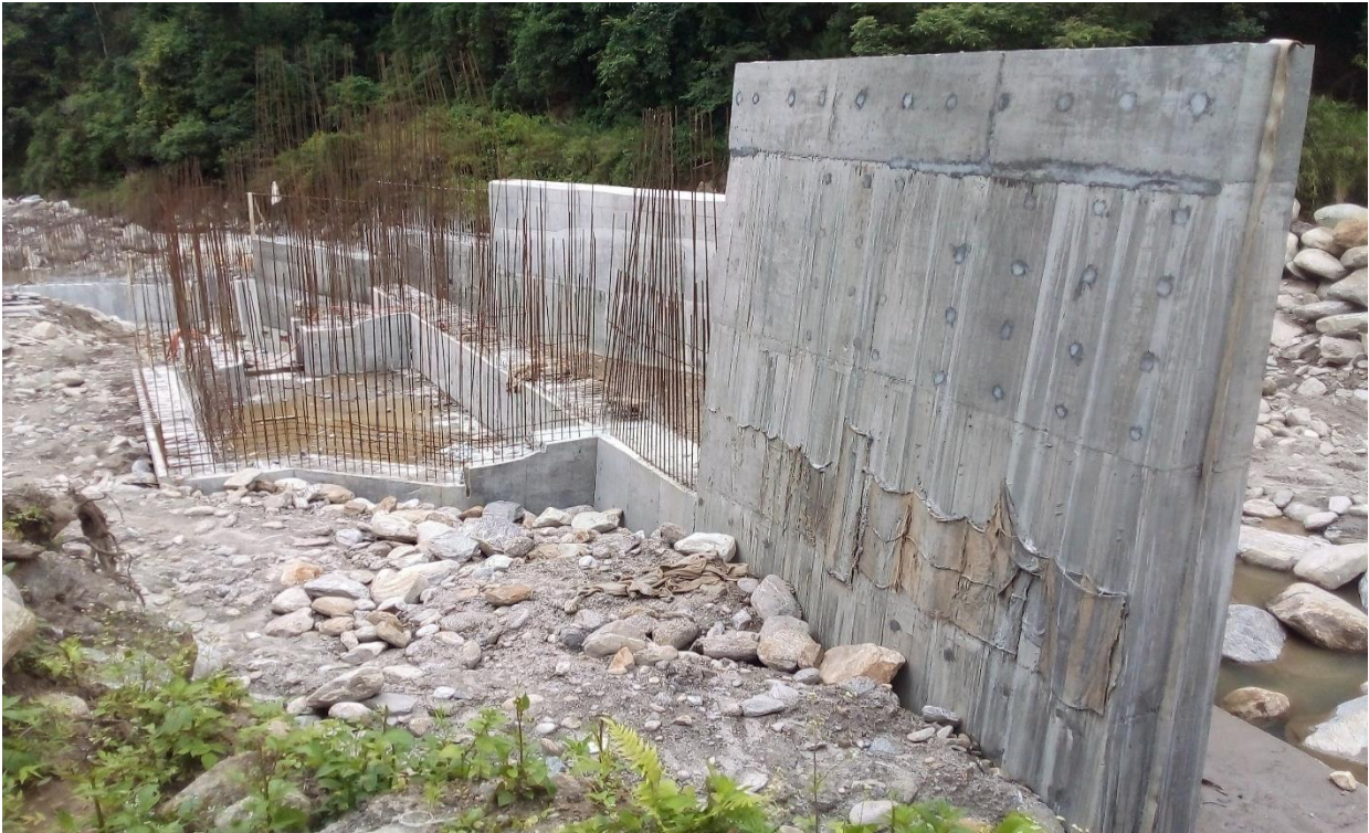
Figure 6.5: Guide wall panel -2 after final concreting.
